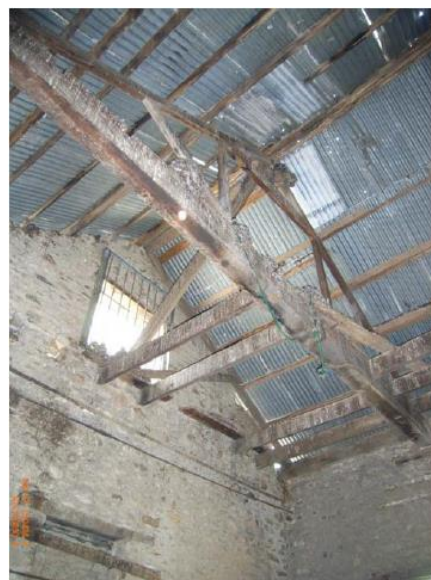
Interior of the mill, showing (left) the south-western space of the ground level, and (right) the north-eastern roof structure with red gum trusses.
