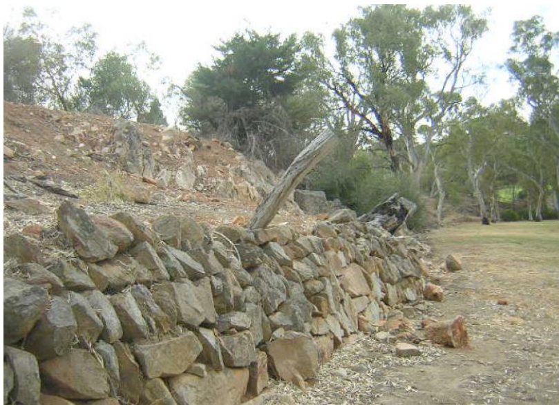
Stone terrace walling along Karrawirra Parri / River Torrens. This was part of the flume system used to convey water from the river to the mill's water wheel.
