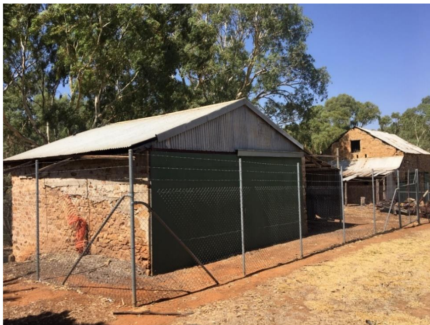
Stone outbuilding north-east of the mill.
